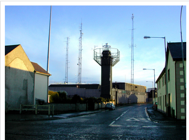
Crossmaglen RUC Barracks, a joint RUC/British Army base built during the operation and demolished in 2007.
